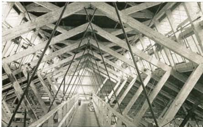
WALK ABOVE MILL FLOOR—SHOWING TRUSS CONSTRUCTION.
