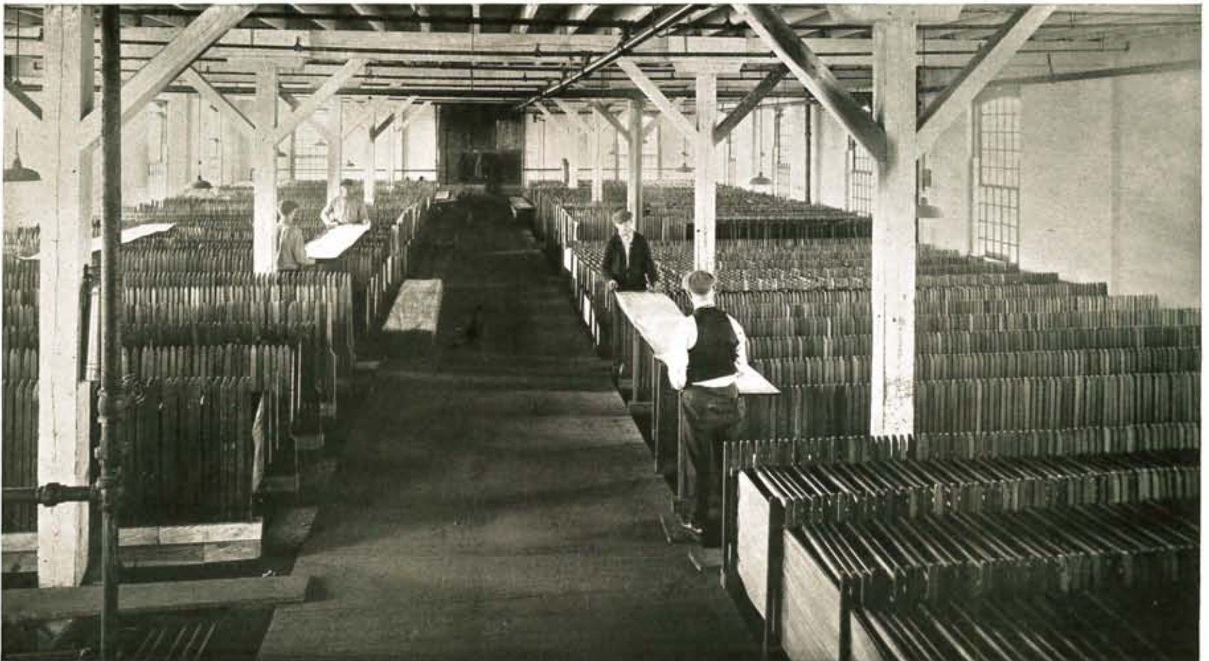
HEAT AND HUMIDITY CONTROLLED VENEER DRYING ROOM.
