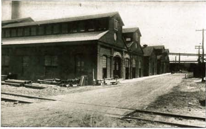
BUILDINGS—G, H AND I—(TURBINE ROOM IN CENTER)
