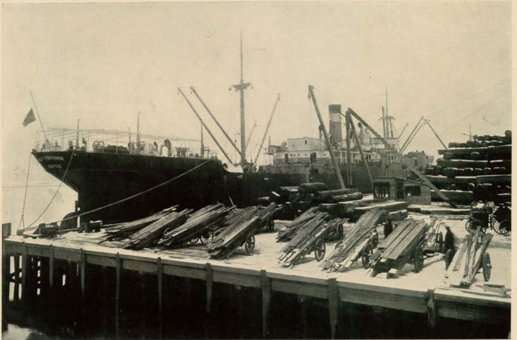
CONCRETE DOCK—350 FEET LONG. 9000 TON S.S. "WEST LOQUASSUCK" FROM AFRICA WITH A FULL CARGO OF 1,000,000 FEET OF MAHOGANY LOGS.
