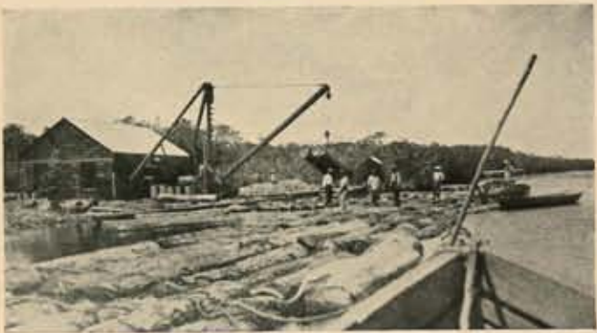
SURVEYING AND MEASURING—USING DERRICK
