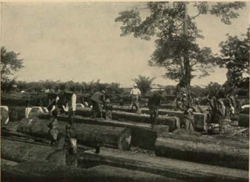
OUR "PLANTATION" FOR THE ACCUMULATION AND STORAGE OF LOGS (Note Railroad Tracks to bring in the logs)
