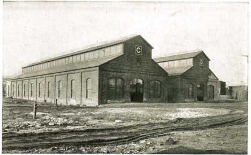
VENEER WAREHOUSES—BUILDINGS C AND D.
