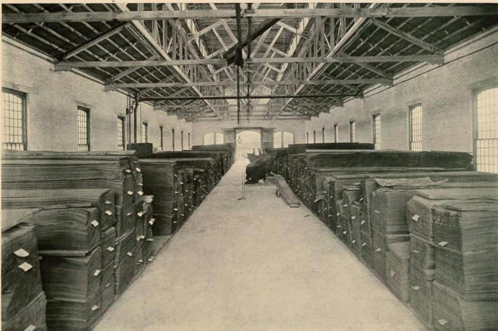
VENEER WAREHOUSE—BUILDING “D”—STORAGE OF SAWN VENEER AND KNIFE CUT 1/20" 1/16" 1/12" 1/10" ETC. ROSEWOOD, SATINWOOD, PADAUK, FRENCH WALNUT, ENGLISH OAK, KOKO, TEAK, ETC.
