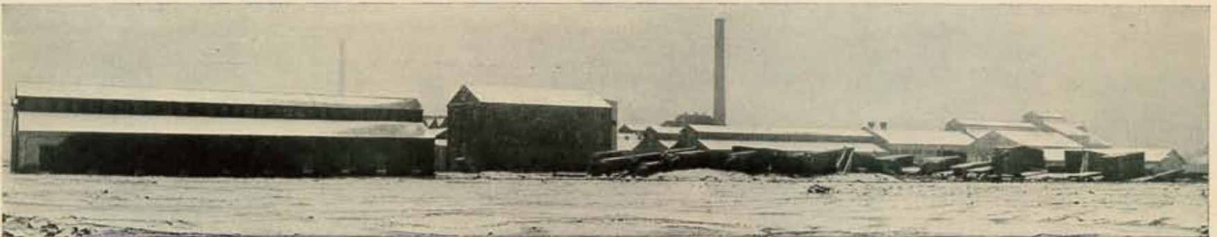
LOWER PLANT—BUILDINGS C-D-E-F-G-H-I-K AND M.—TAKEN JUST AS CONSTRUCTION WAS COMPLETED.
