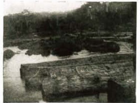
RIVER BED—NEARLY DRY
