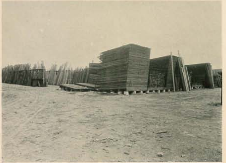
CAREFULLY PILED LUMBER—FIVE BEARING FOUNDATIONS.
