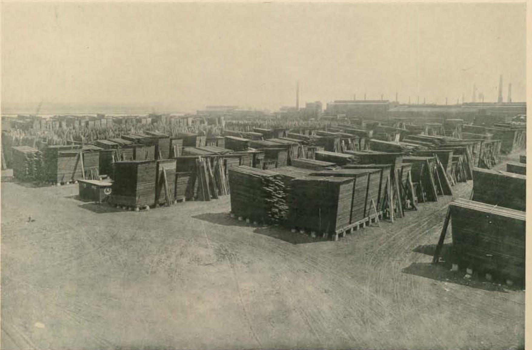
GENERAL VIEW OF SOUTH CORNER OF THE LUMBER YARD. ( all Mahogany in view. )
