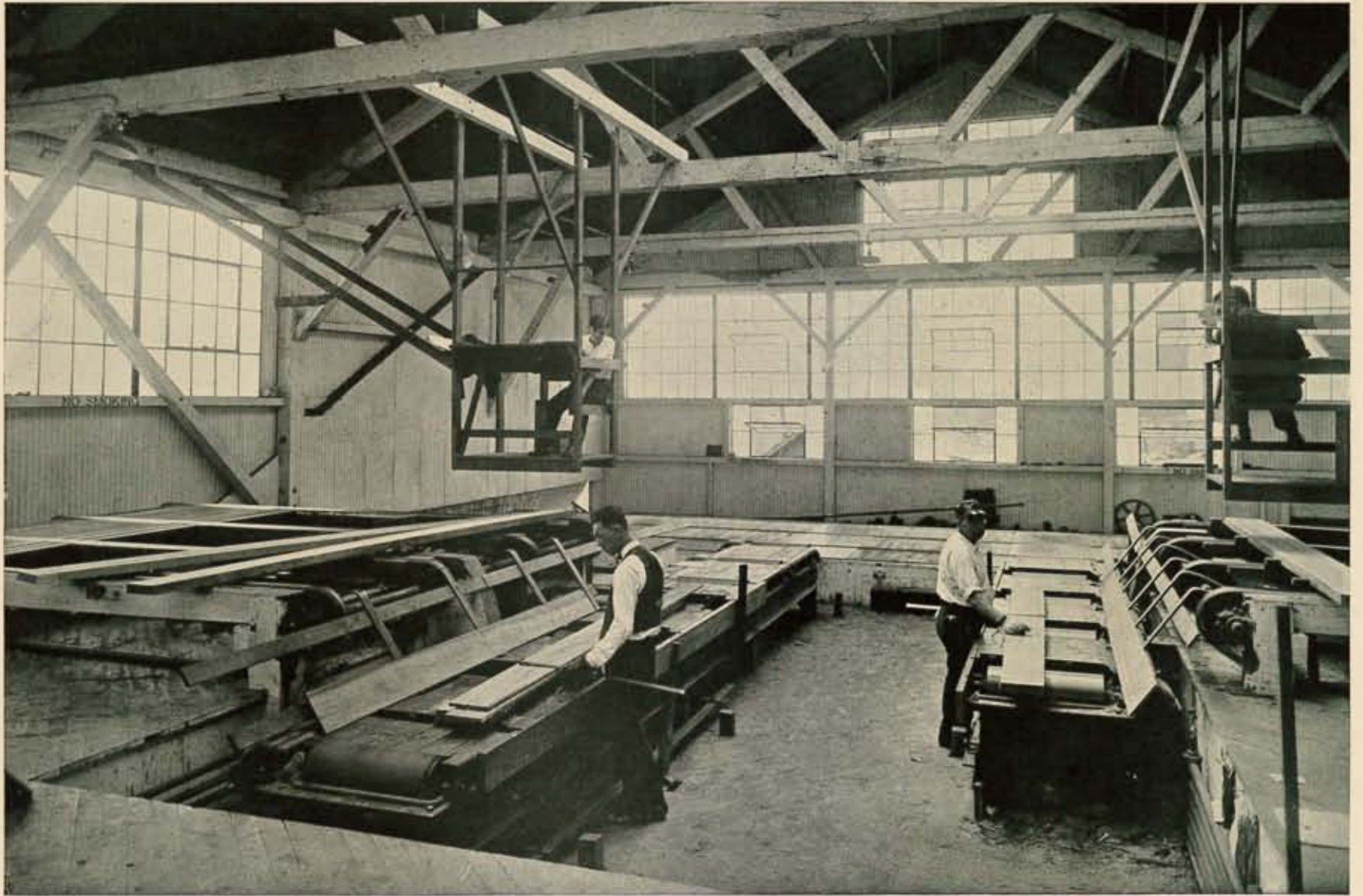
INSPECTION ROOM—(Note the abundance of light—the tally boys in stations directly over the tables.) THE ARRANGEMENT OF TABLE FEED CONTROL WITH LUMBER COMING TO THE INSPECTOR on edge IS AN INNOVATION IN INSPECTION. A PRESSURE OF FOOT ON FLOOR ROD, REMOVES THE LUMBER, SENDING IT ON OUT TO THE SORTING TABLE.
